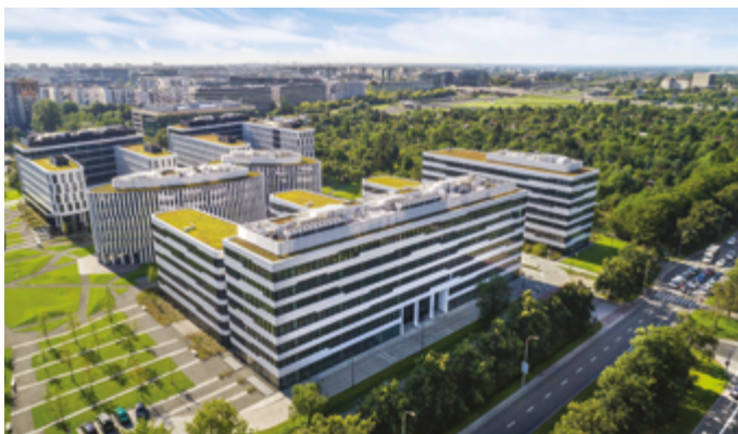
Business Garden Warsaw, Warszawa, Poland, Certification level: Platinum 2017
